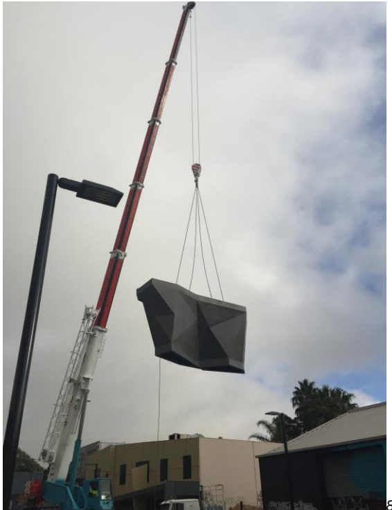
May 2015 , the bouldering wall is lowered into place
